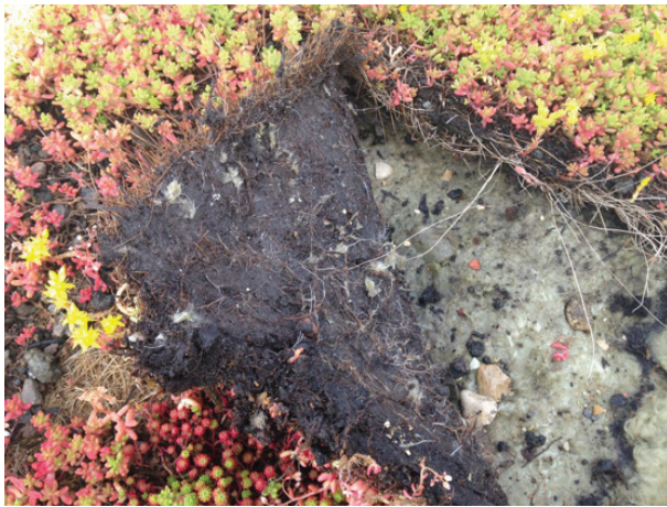
Mini rooting of the vegetation into Urbanscape® green roll after one week.
